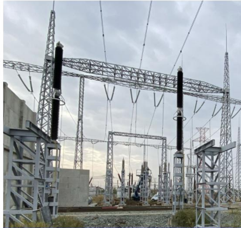
Civil and electrical works
