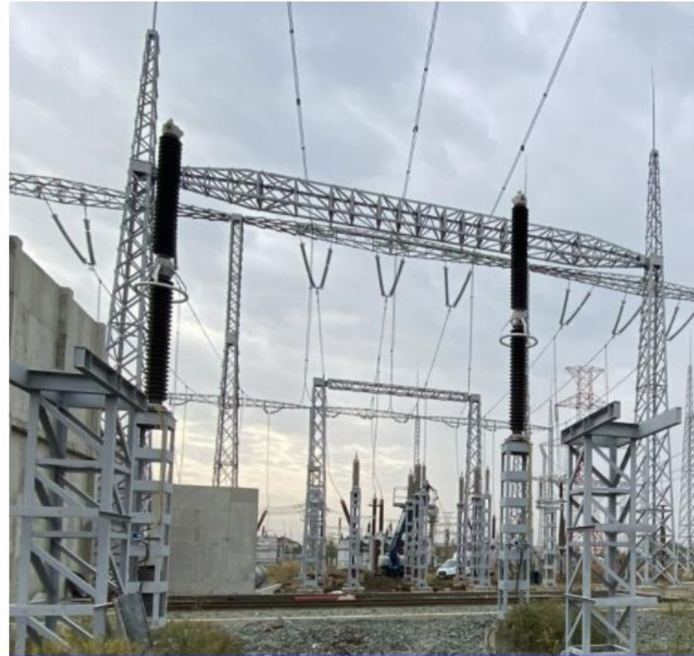
Civil and electrical works
